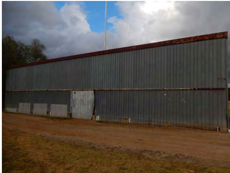
Photo 2 – view of grandstand from rear (Binalong Street façade)
