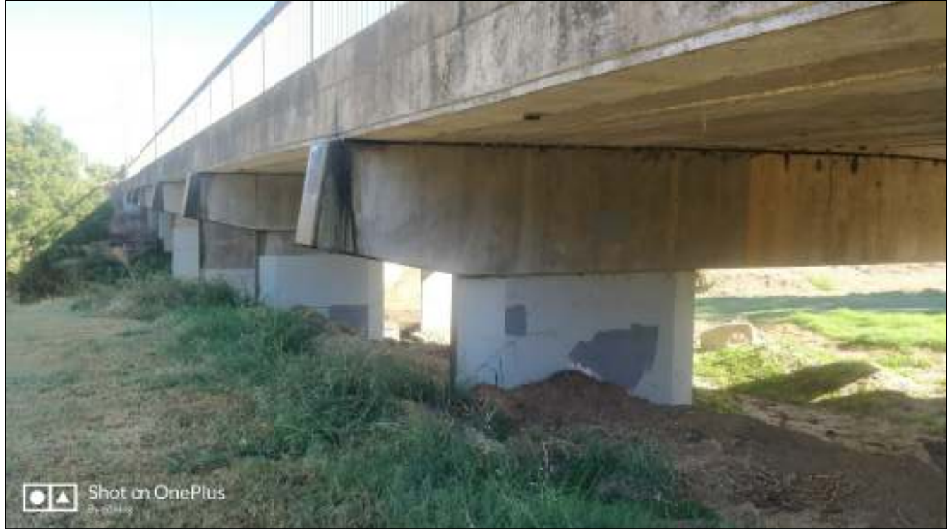
Flood Mark 1 – Bridge Support Beam
