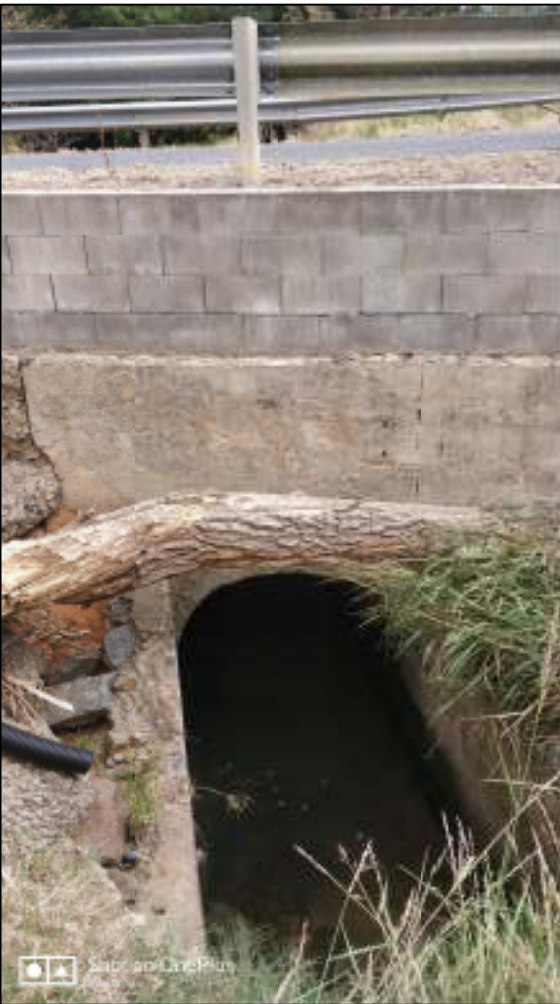
Culvert Woolrych Street - upstream side
