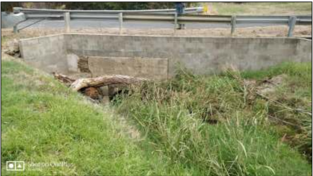
Culvert Woolrych Street - upstream side
