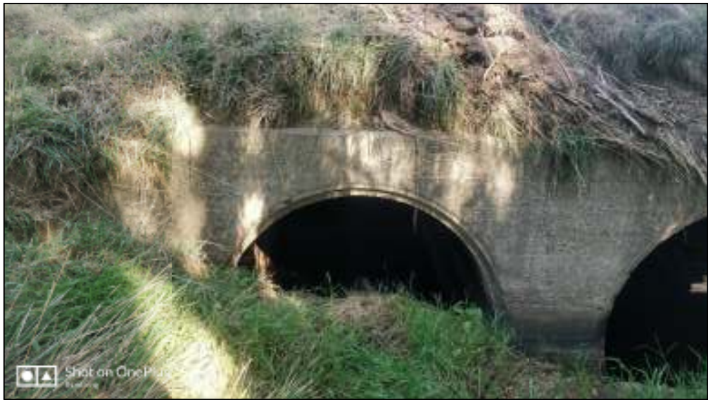
Culvert Aurville Road – upstream side Southern end
