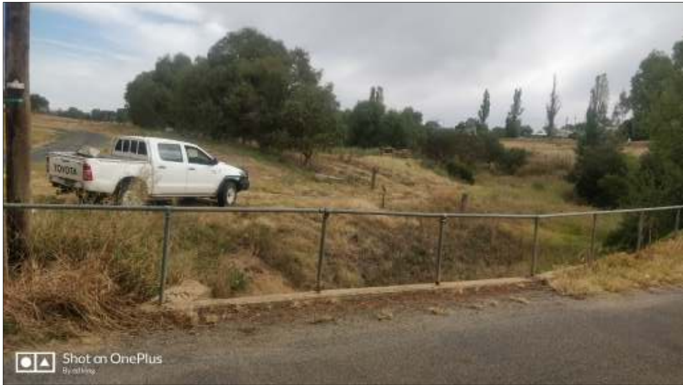
Vernon Street Bridge - looking upstream from bridge
