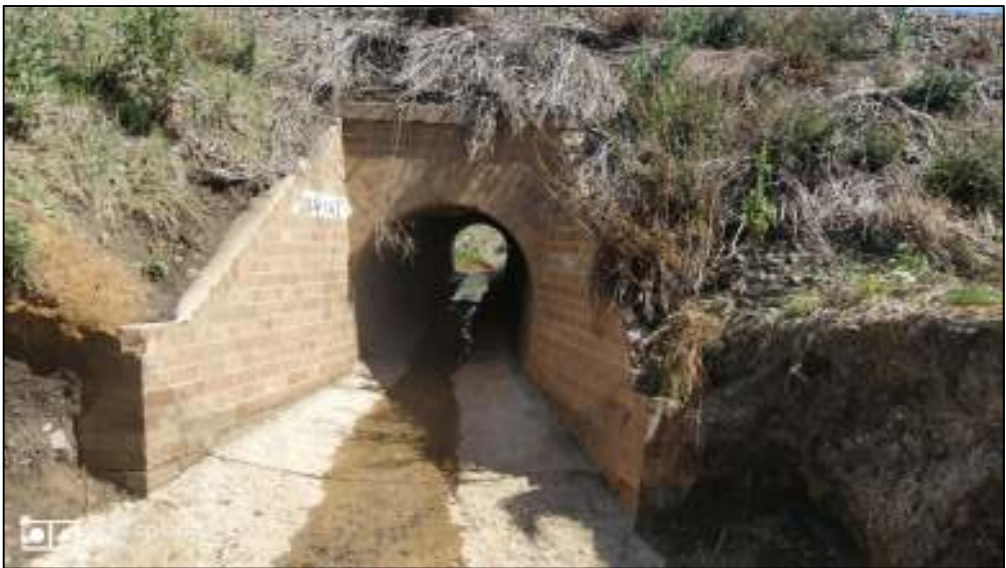
Culvert Small Rail 03 - downstream side
