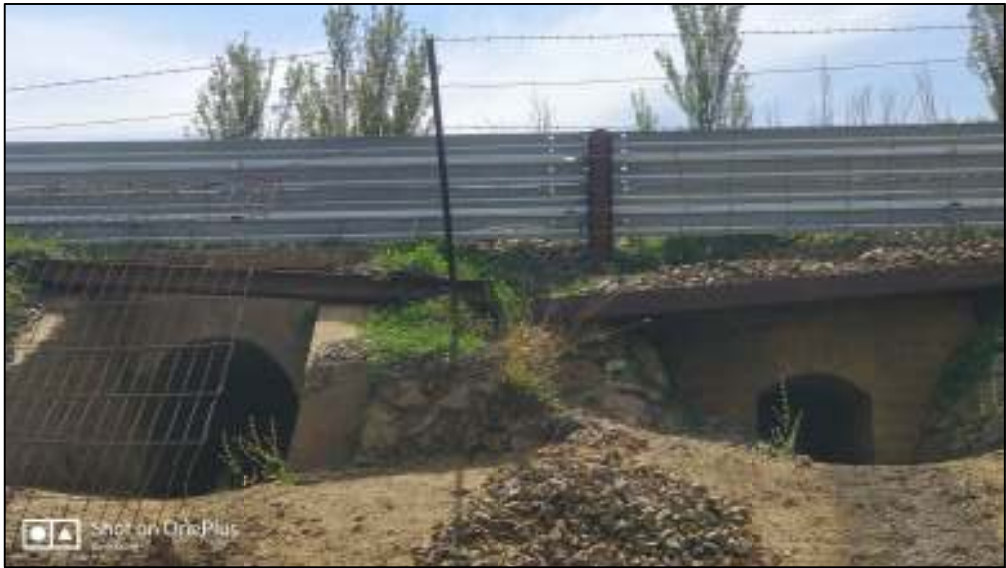
Culvert Rail 02 - downstream side
