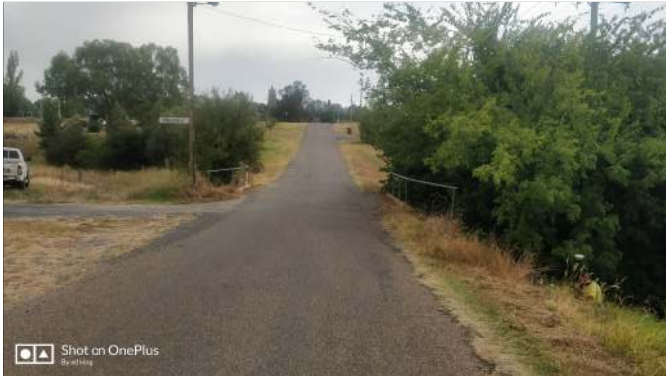
Vernon Street Bridge - looking north across bridge
