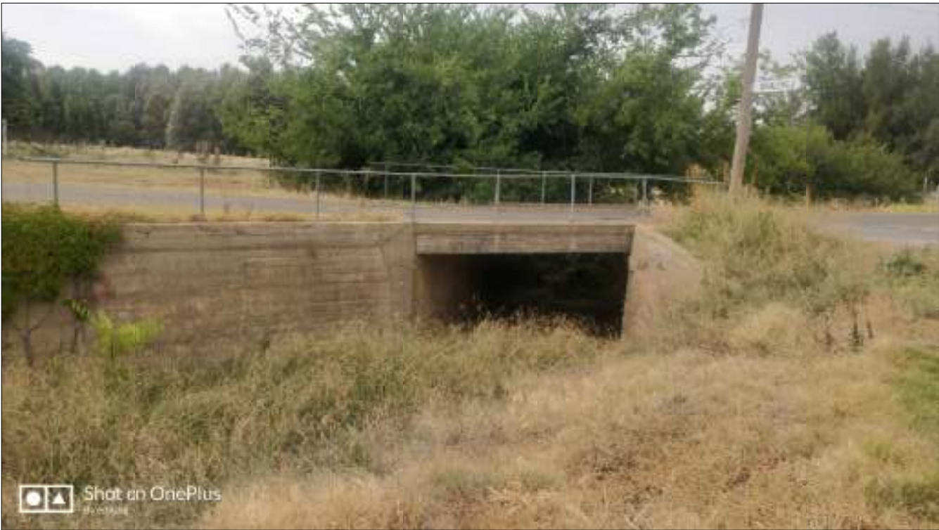
Vernon Street Bridge - looking downstream
