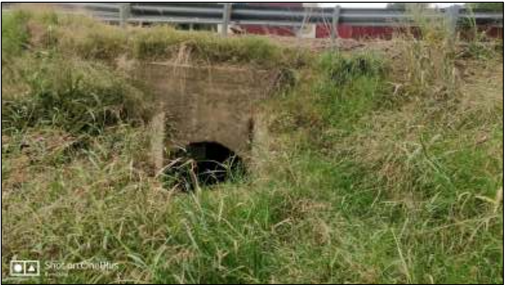
Culvert Woolrych Street - downstream side
