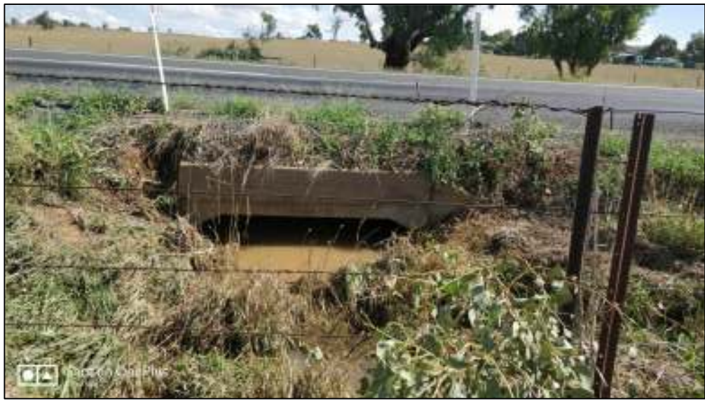
Culvert Road 01 - downstream side
