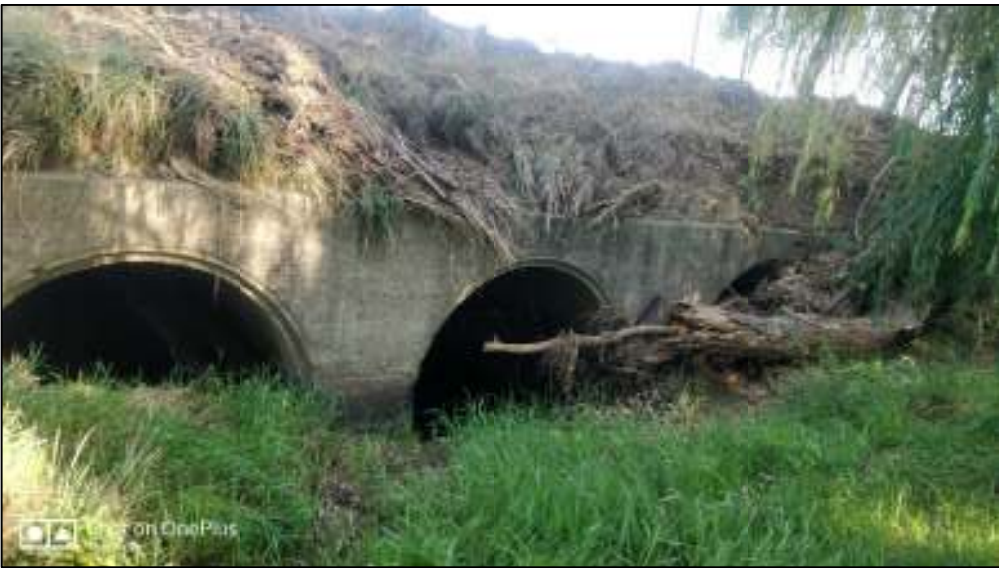
Culvert Aurville Road – upstream side Northern end
