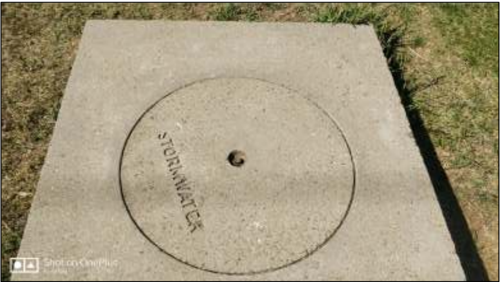
Culvert Ward Street - lid on the likely pipe alignment
