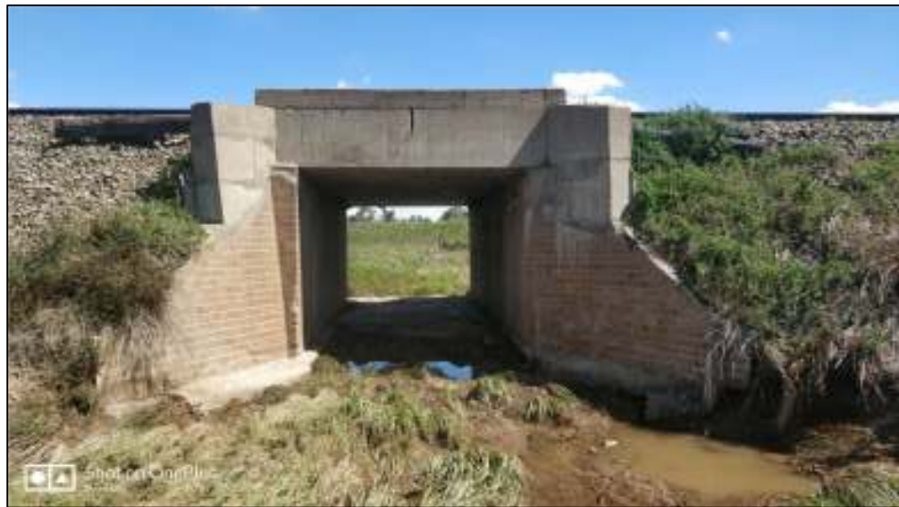
Culvert Small Rail 04 - downstream side
