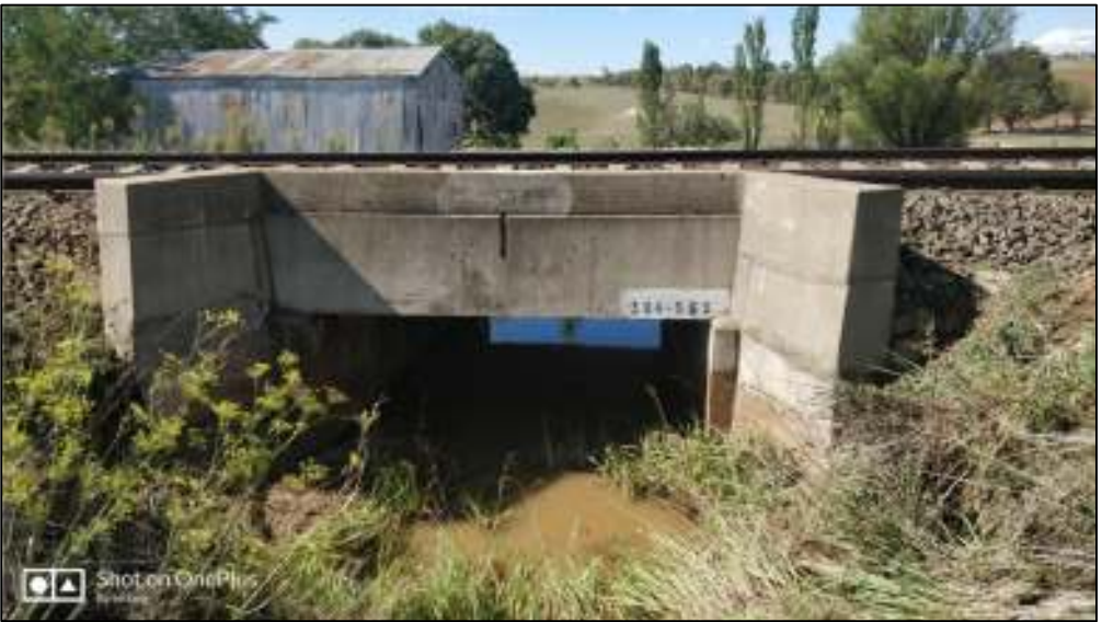
Culvert Small Rail 02 - upstream side
