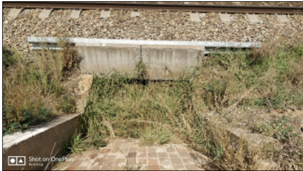
Culvert Rail 01 - upstream side
