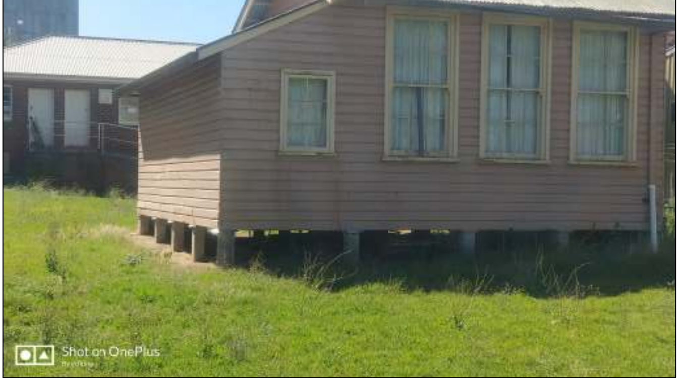
Flood Mark 4 – Demountable building
