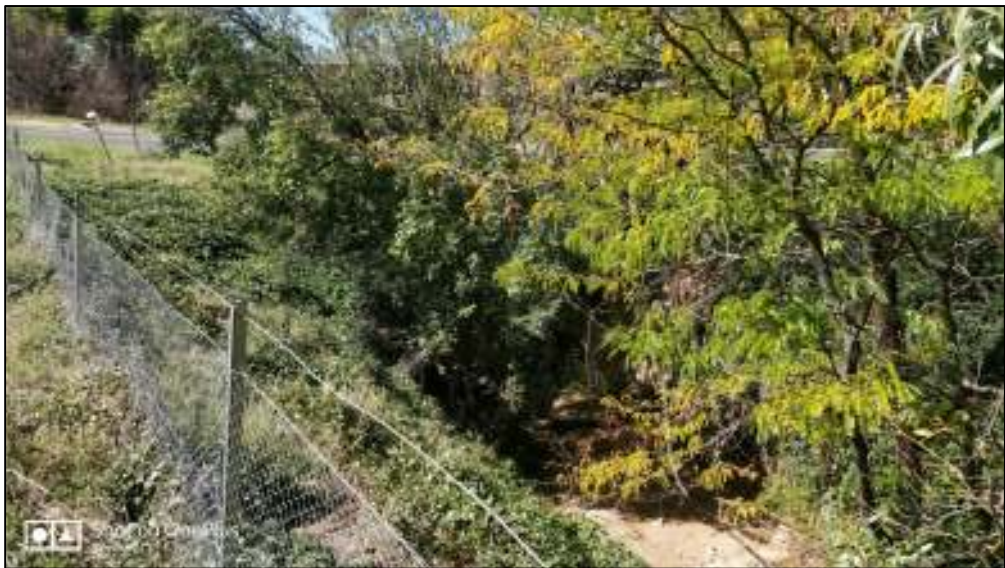
Culvert Ward Street - downstream side
