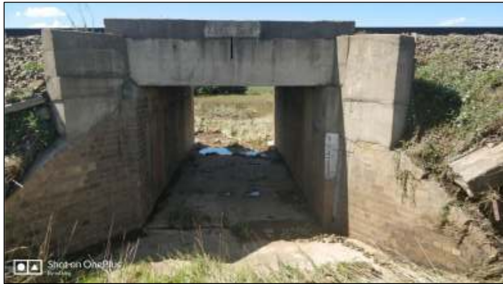
Culvert Small Rail 04 - upstream side
