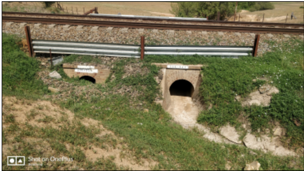
Culvert Rail 02 - upstream side
