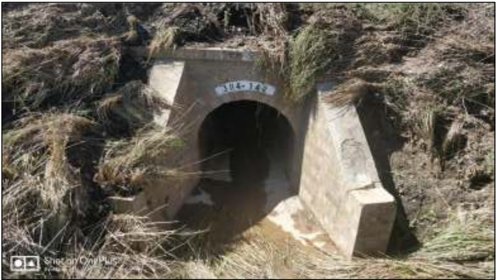
Culvert Small Rail 03 - upstream side
