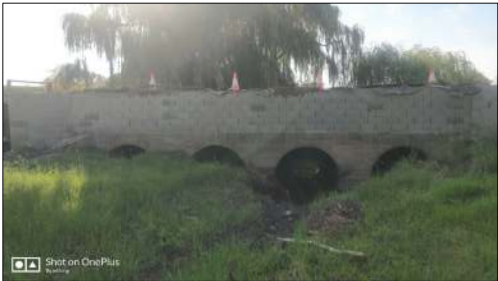
Culvert Aurville Road – downstream side
