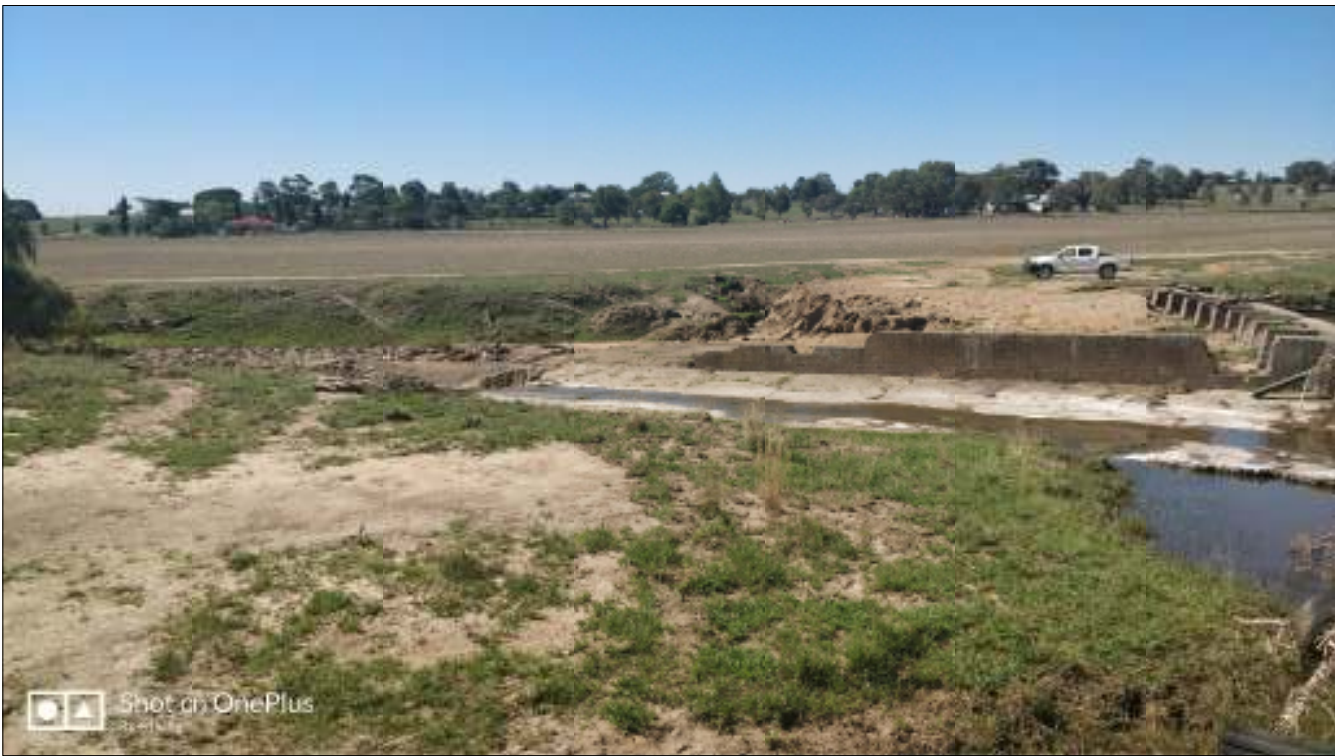
Weir 02 - looking North from bank
