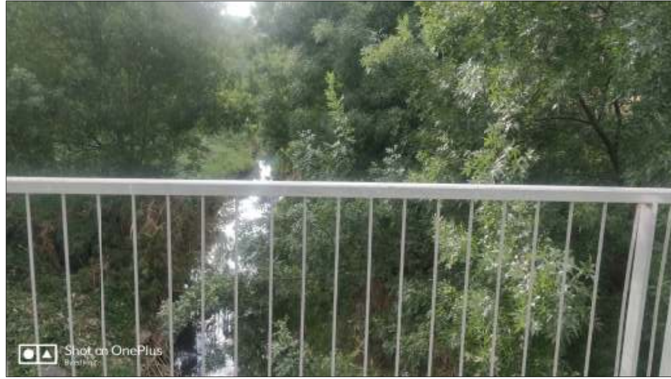
Bathurst Street Bridge - looking upstream from bridge
