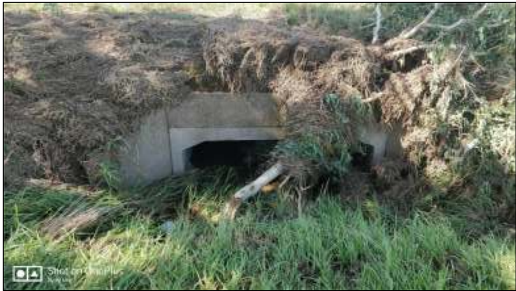
Culvert Road 01 - upstream side
