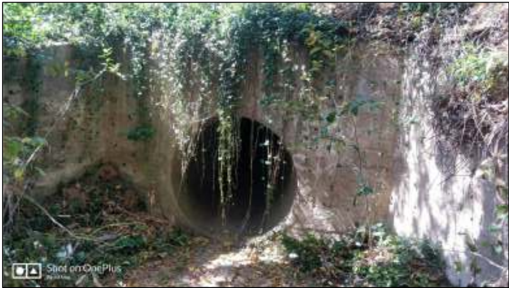
Culvert Ward Street - downstream side
