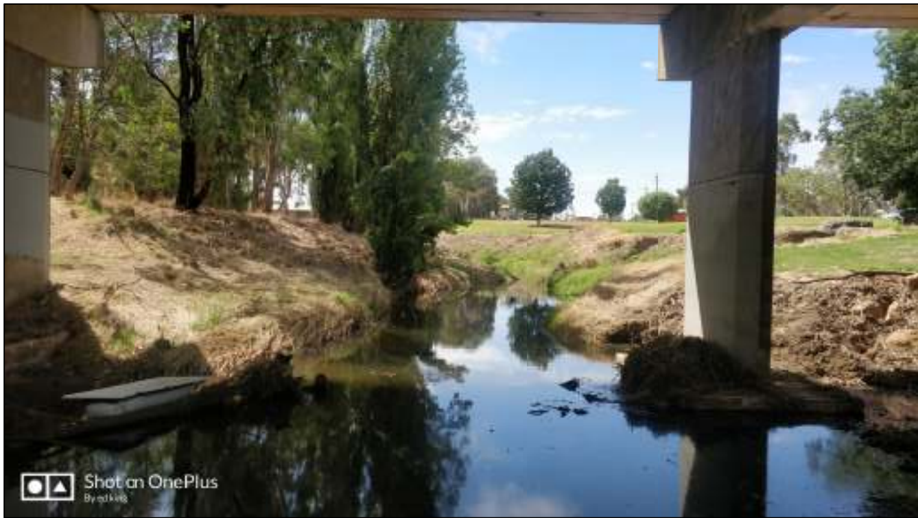
Albury Street Bridge - looking upstream
