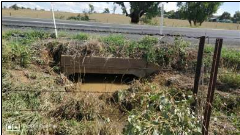
Culvert Road 01 - downstream side
