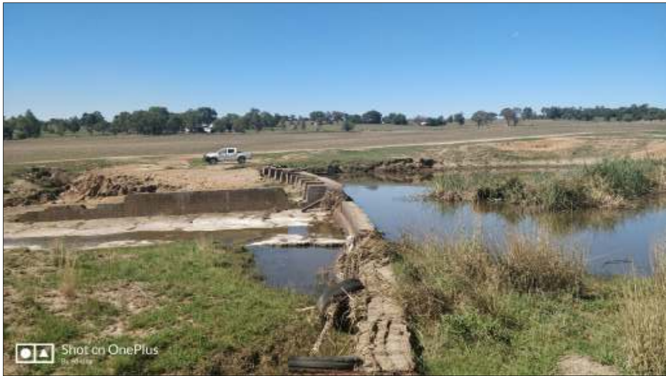
Weir 02 - looking North from bank
