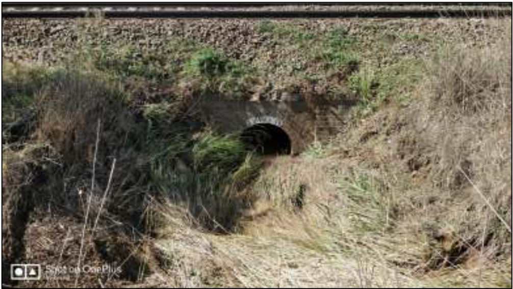
Culvert Small Rail 01 - upstream side
