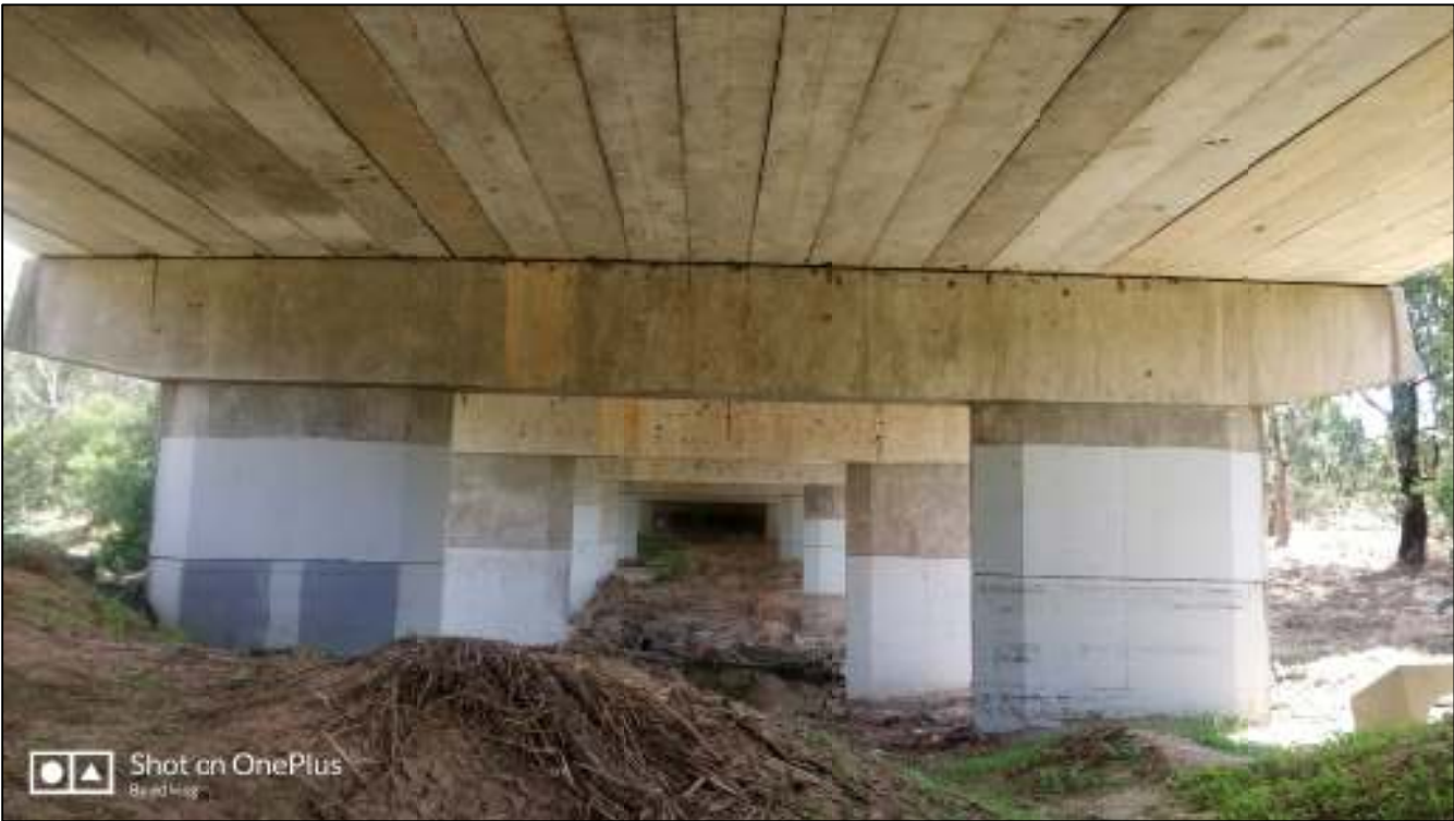
Albury Street Bridge - structure looking West
