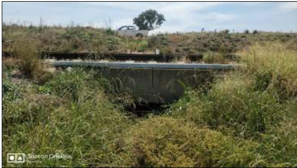
Culvert Rail 01 - downstream side
