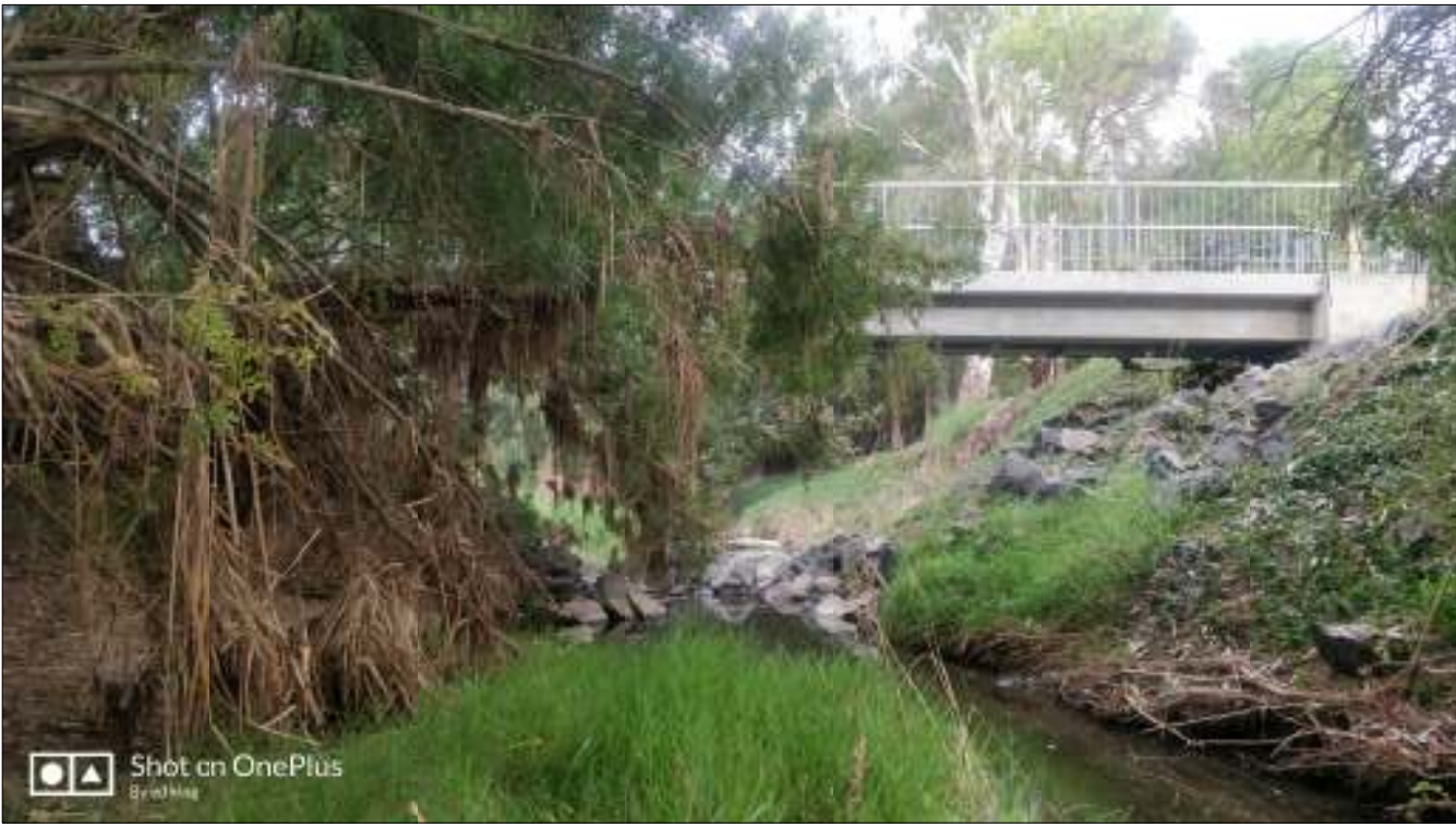
Bathurst Street Bridge - looking downstream
