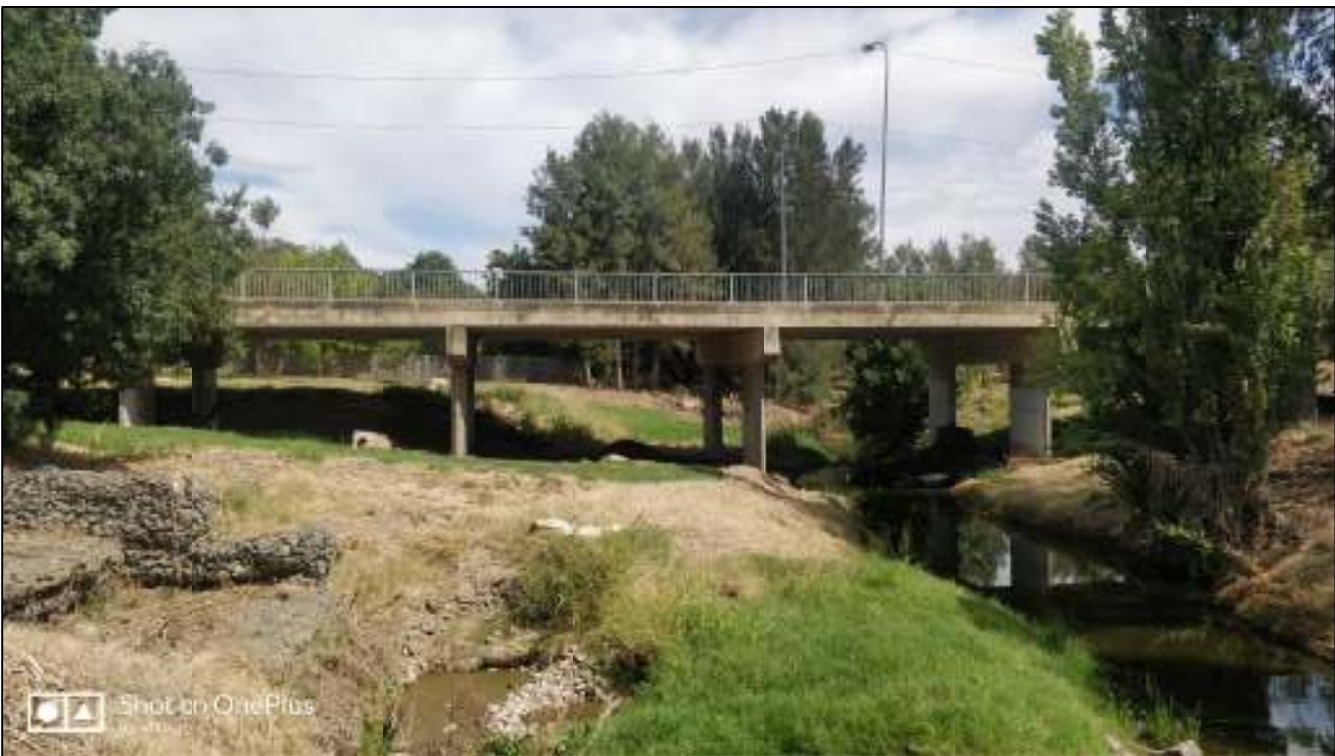
Albury Street Bridge - looking downstream
