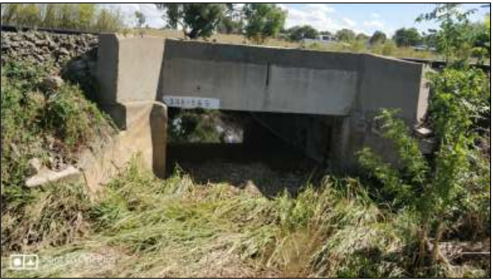
Culvert Small Rail 02 - downstream side
