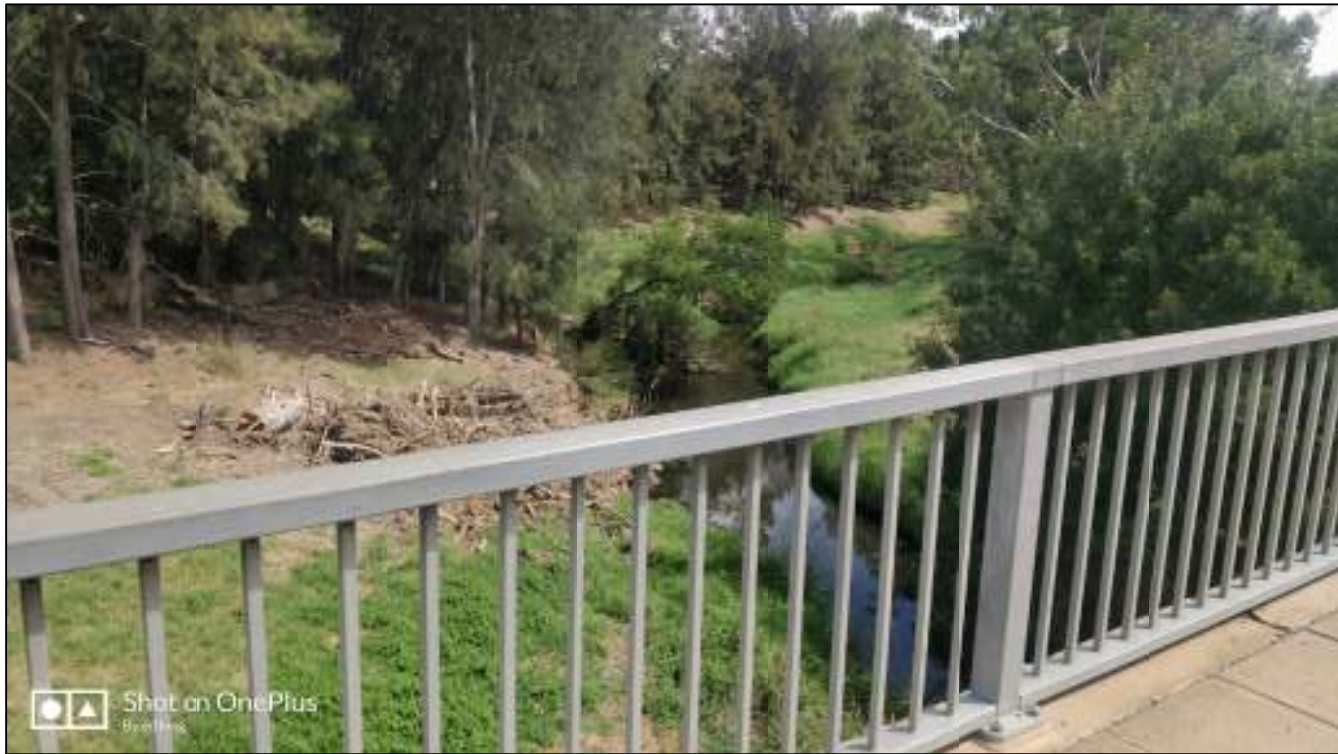
Albury Street Bridge - looking downstream from bridge
