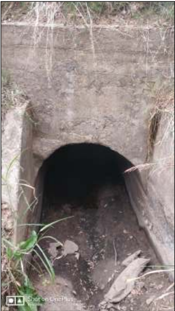
Culvert Woolrych Street - downstream side
