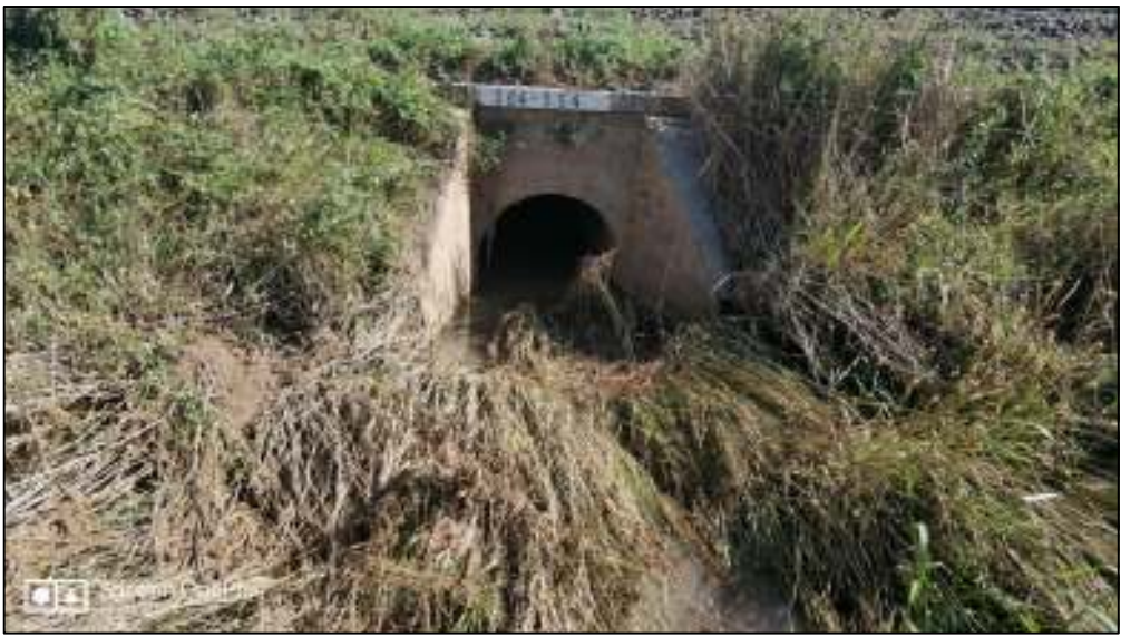
Culvert Small Rail 01 - downstream side
