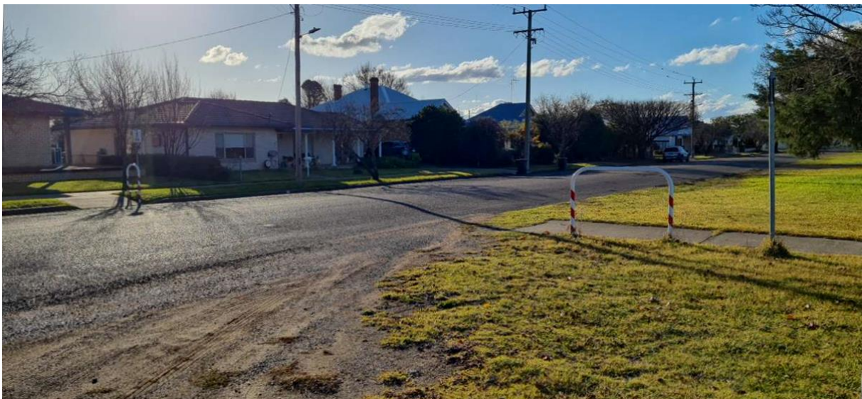
Figure 3.35 Footpath near Boorowa Recreation and Bowling Club with no separation between road and footpath level
