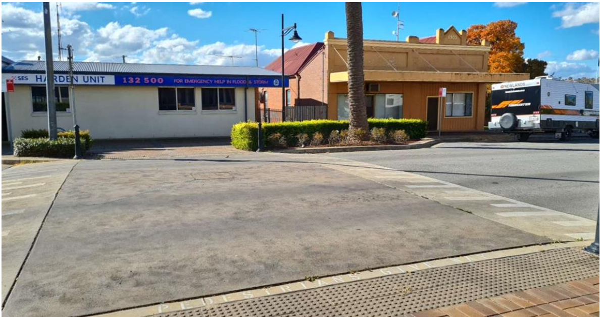
Figure 3.30 Raised pedestrian crossing in Harden town centre with vehicle priority
