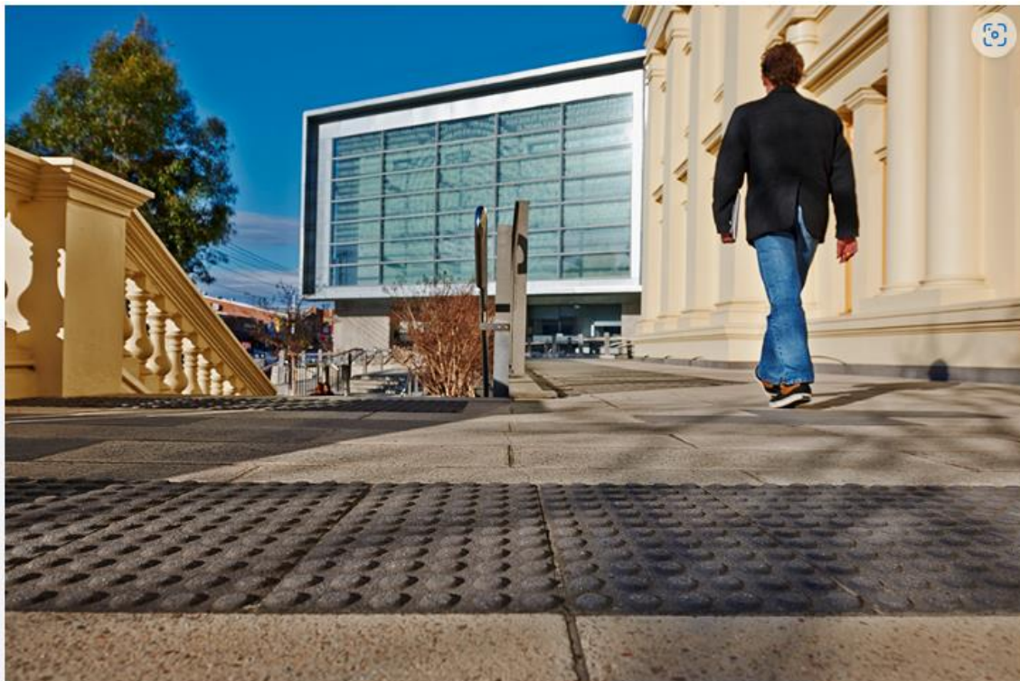
Figure 4.4 Tactile Ground Surface Indicators example (TGSIs)
