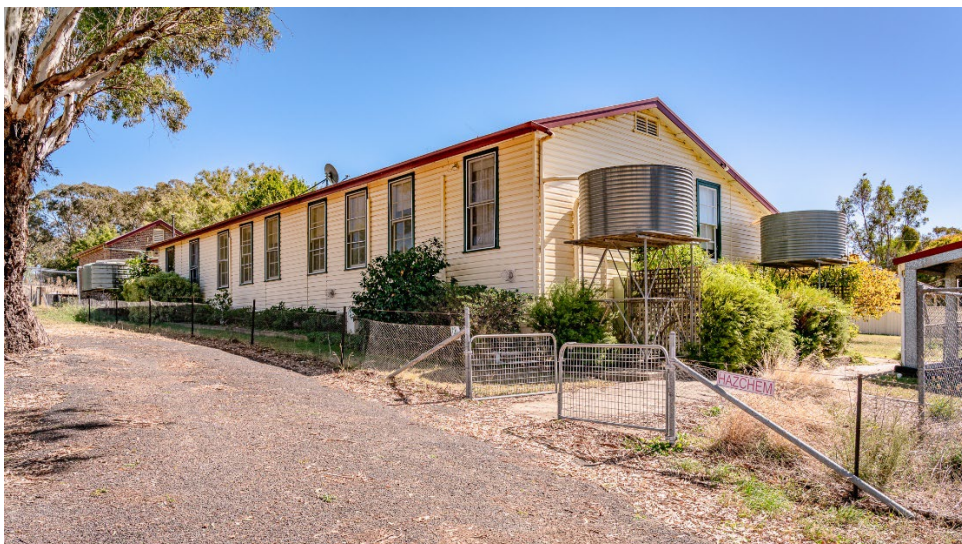
Rye Park Public School. Image courtesy of Greg Davis.
